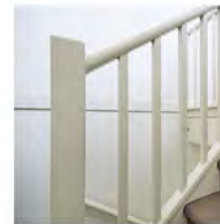
a. Timber Handrail with Timber Balustrade
